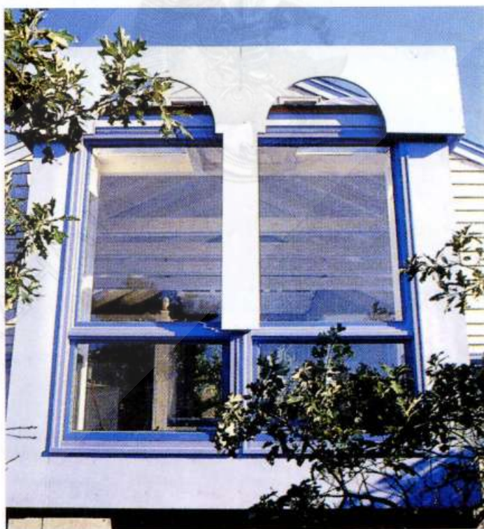
Είχ. 19. Ἐπαγγελματικός χώρος ἀπὸ τὸν Charles Jencks (JENCKS, The Language of Post-Modern Architecture )
