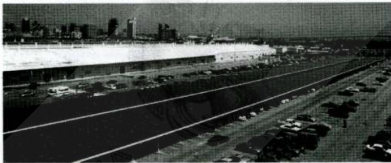
Figure 3-5: U.S. Navy 750 kW Parking Lot Solar PV Installation Near San Diego
