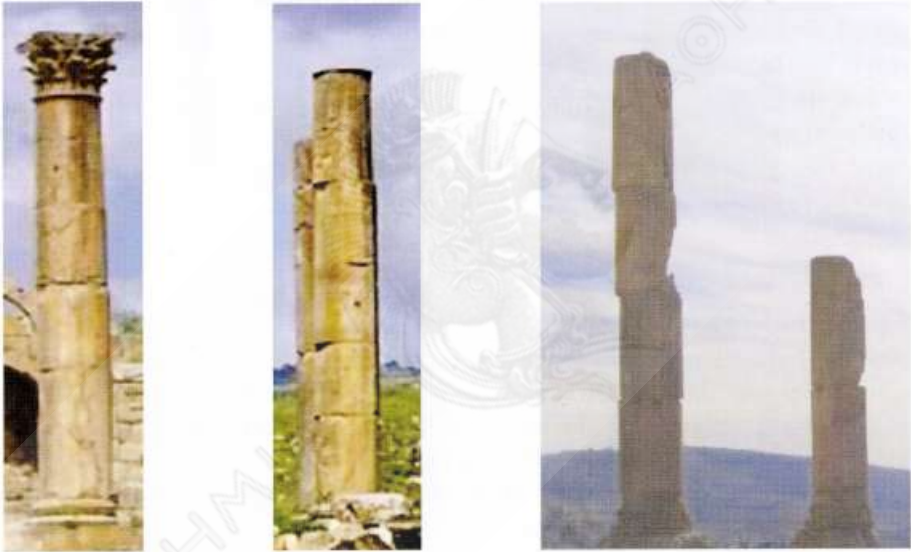
Fig. [35]: A contre-lumière view of columns in Jerash, showing the loss of stone due to rocking. The movement of these columns can be seen today by wedging a twig between the drums and watching it move up and down as the column sways.
