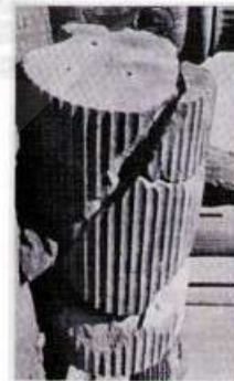
Fig. [4]: Diagonal cracks of drums.
