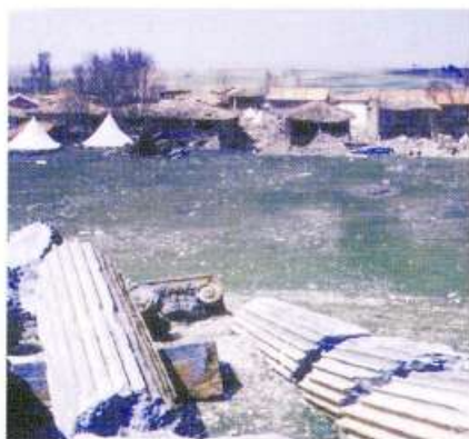
Fig. [8]: Fracture of toppled monolithic columns caused by the earthquake of 1970. In the background can be seen the ruined village of Çavdarhisar.
