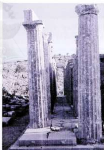
Fig. [24]: A solitary column, next to the missing column of the south colonnade, leaning by 17 cm to the south in 1965.
