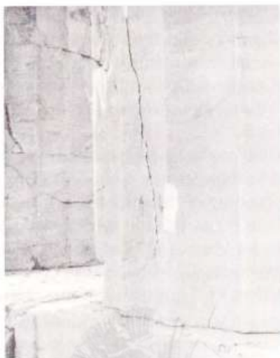
Figure [57]: First drum (anathyrosis) of the NE column of Parthenon after the earthquake of 1981 showing incipient right-lateral shear failure most probably due to rocking.
