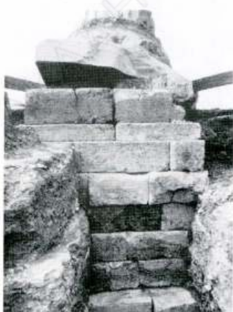
Fig. [38]: A view of the column blown down in 1852, which most probably fell owing to failure of its base plinth.
