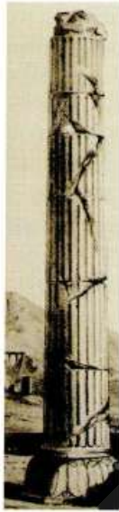
Fig. [1]: Damaged column in Persepolis.
