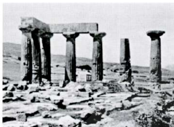
Fig. [32]: A view of the temple from the east after it had been excavated in 1927.
