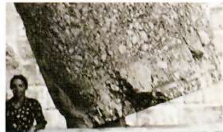
Fig. [22] The final position of the column of the south peristyle of the Temple of Bacchus, showing the crashed edge of its bottom drum resting on the stylobate (1968).
