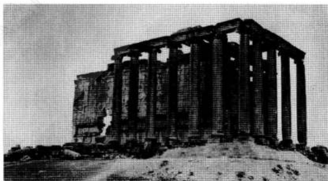
Fig. [7]: The Temple of Zeus after the earthquake of 1970, which caused the collapse of the three columns shown standing on the left of the temple in Figure [6].
