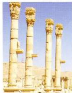
Fig. [42]: Pillars of the colonnade with statue brackets in Palmyra, Tadmor. Most of the upper drums are dented at the edge.
