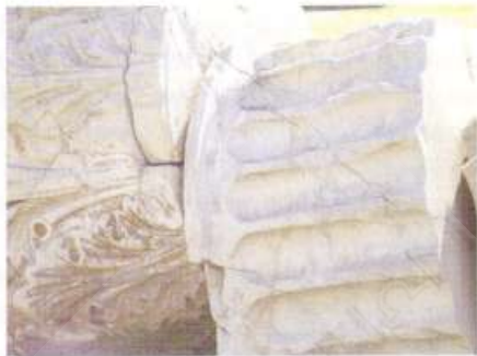
Fig. [41]: The first drum under the capital of the column of Olympieion Zeus in Athens blown down in the storm of 1852, showing a diagonal trace of incipient failure.
