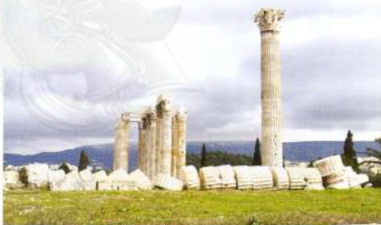
Fig. [38]: A view of the column blown down in 1852, which most probably fell owing to failure of its base plinth.
