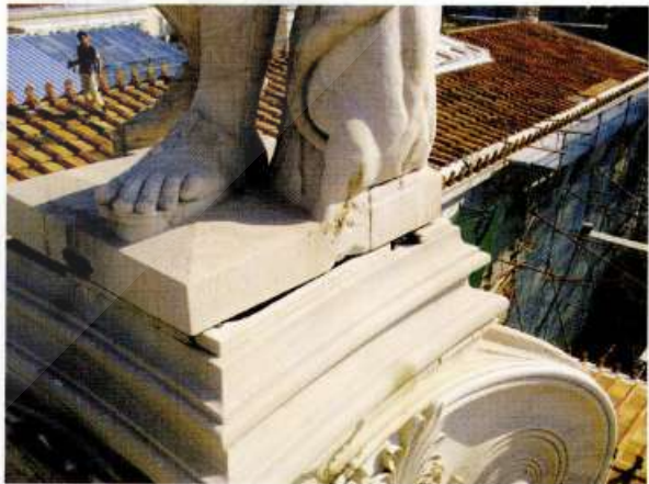
Fig. [18]: Displacement and rotation of statue caused by the earthquake of 1999.
