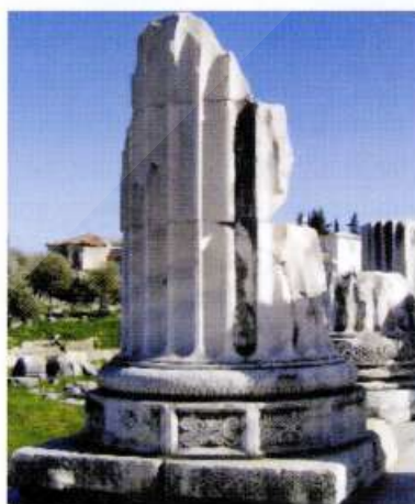
Fig. [33]: The stump of a column that failed in shear.
